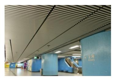
Durlum Tubular - Linear flow open concept tubular metal ceiling
