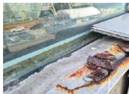
Figure 15.3: Standard galvanized coatings showing significant deterioration (located within close proximity to the coastline)
