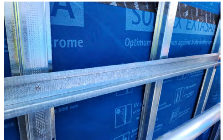
Figure 18.3: Sarking complete with top hat subframe
