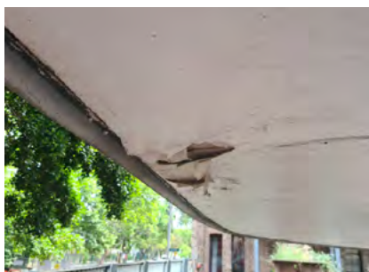
Figure 15.5: Inadequate weatherproofing resulting in moisture ingress
