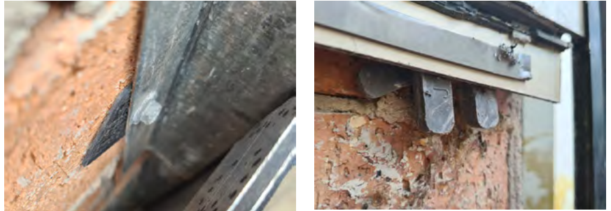
Figure 15.8: Combustible components (packers)
