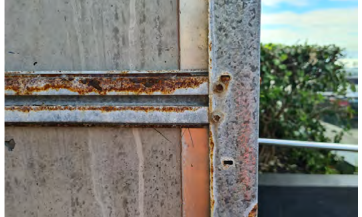
Figure 5.5: Care must be taken with products formed from galvanized sheet to prevent corrosion
