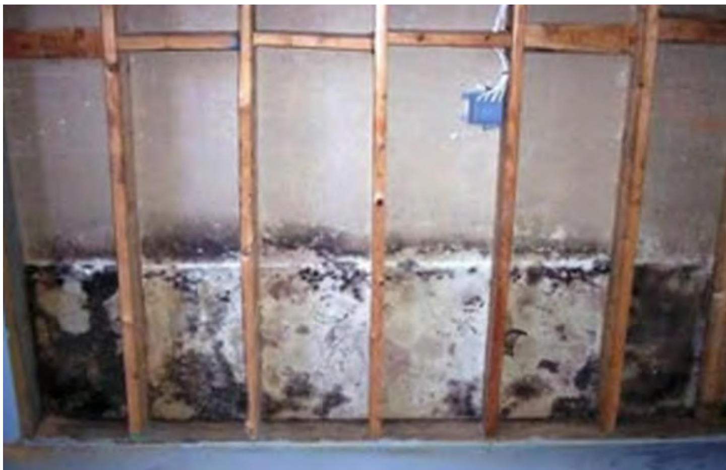
Figure 11.1: Black mould growth in a wall cavity due to poor ventilation and condensation on inside face of cladding
