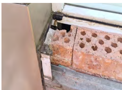
Figure 15.6: Inadequate wall structure
