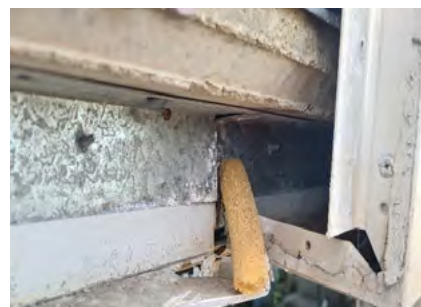
Figure 15.4: Inadequate fixings of subframing to supporting structure
