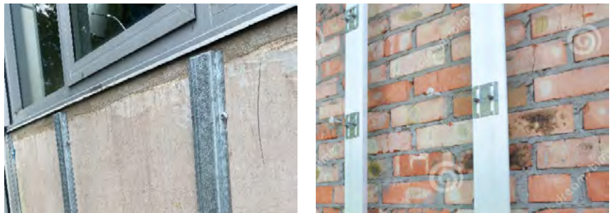
Figure 15.9: Inadequate or lack of insulation
