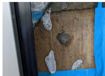
Figure 15.5: Inadequate weatherproofing resulting in moisture ingress
