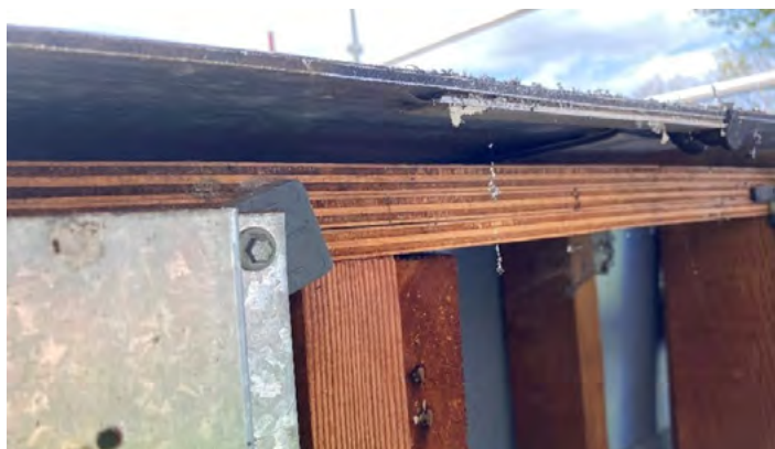
Figure 18.7: Timber parapet framing
