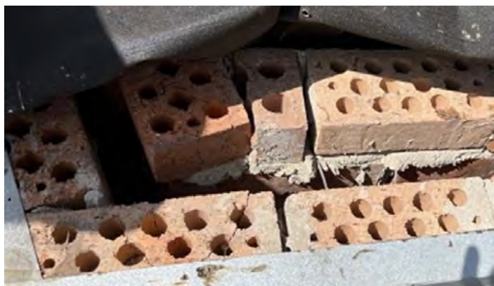
Figure 18.5: Defective masonry construction
