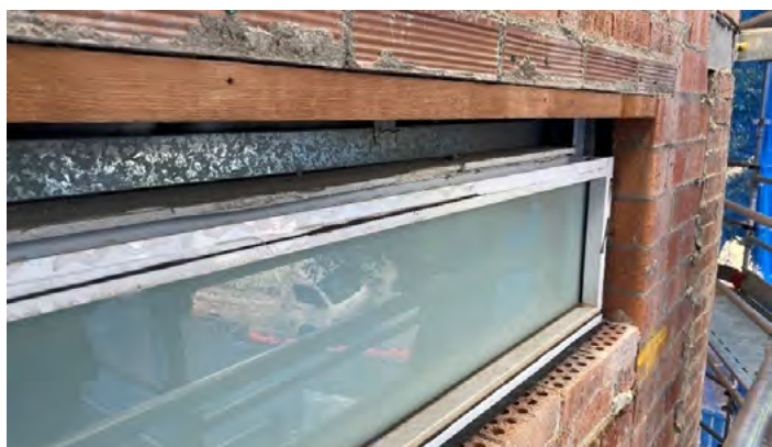
Figure 18.6: Timber lintels
