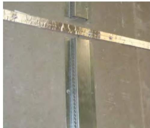
Figure 10.6: Cavity barriers are to be continuous
