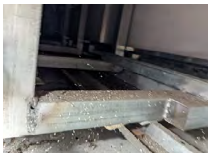
Figure 15.4: Inadequate fixings of subframing to supporting structure
