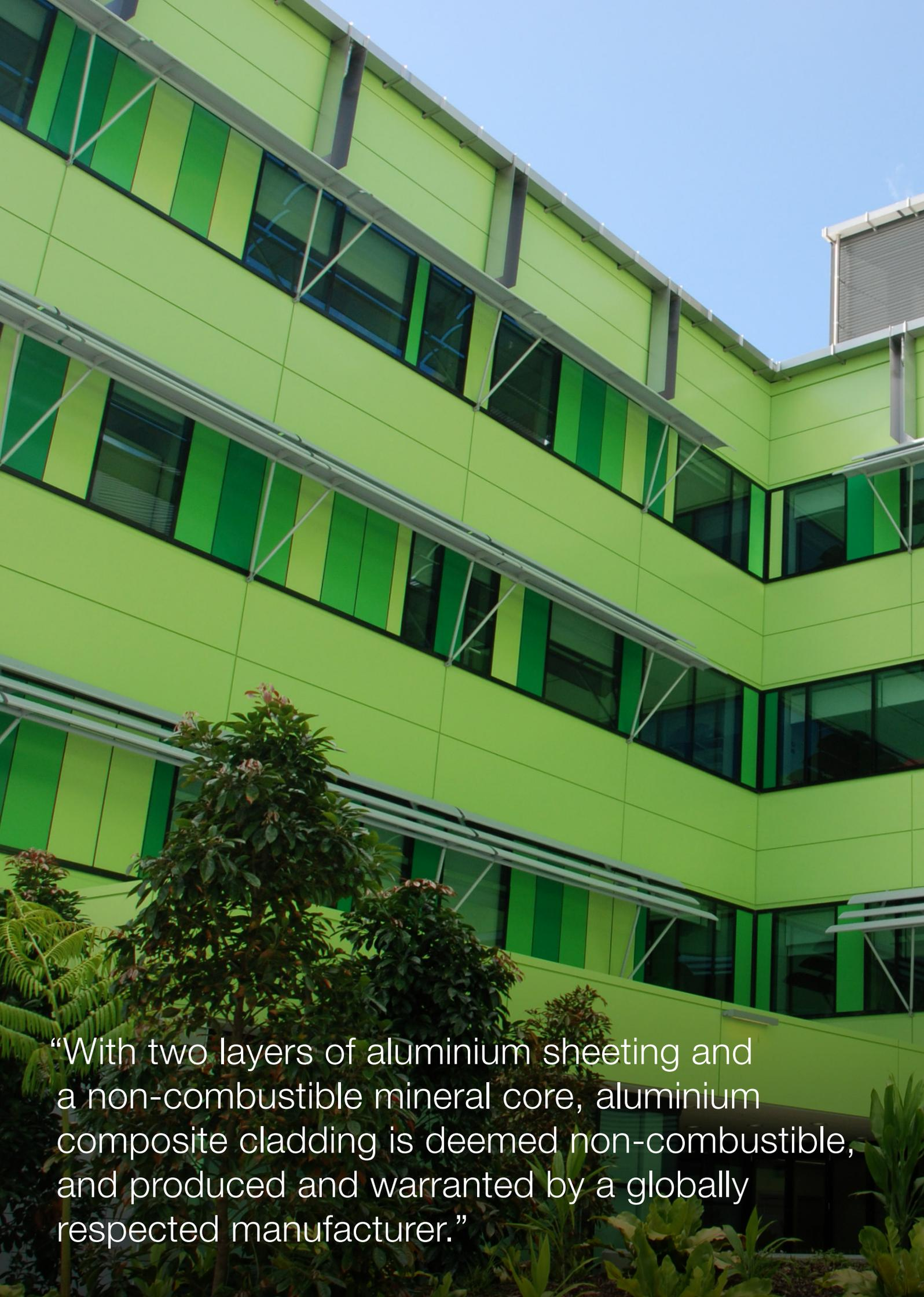
“With two layers of aluminium sheeting and a non-combustible mineral core, aluminium composite cladding is deemed non-combustible, and produced and warranted by a globally respected manufacturer.”
